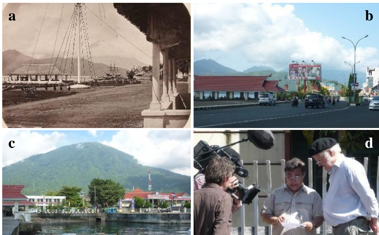
Figure 2: Dutch colonial administration center of Ternate. (a) Resident's Pier, built in 1811, as seen in 1880 (University of Leiden, KITLV Digital Image Library). The pier had undergone several renovations and collapsed in 1963. (b) The Resident's Pier in 2009, following renovation in 1996 by the North Maluku Regency in partnership with PT Semana Graha Geovani. (c) View of Ternate from the pier. (d) One of us (SM), with de Clercq's map in hand, explaining our strategy to locate Wallace's Ternate house to Redmond O'Hanlon, British writer and scholar, during the production of a program on Alfred Russel Wallace by VPRO, 3–9 June 2009.
